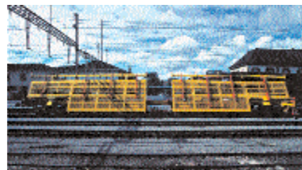
External preassembly of the switch
