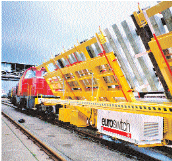
Just-in-Time delivery on the day of installation
